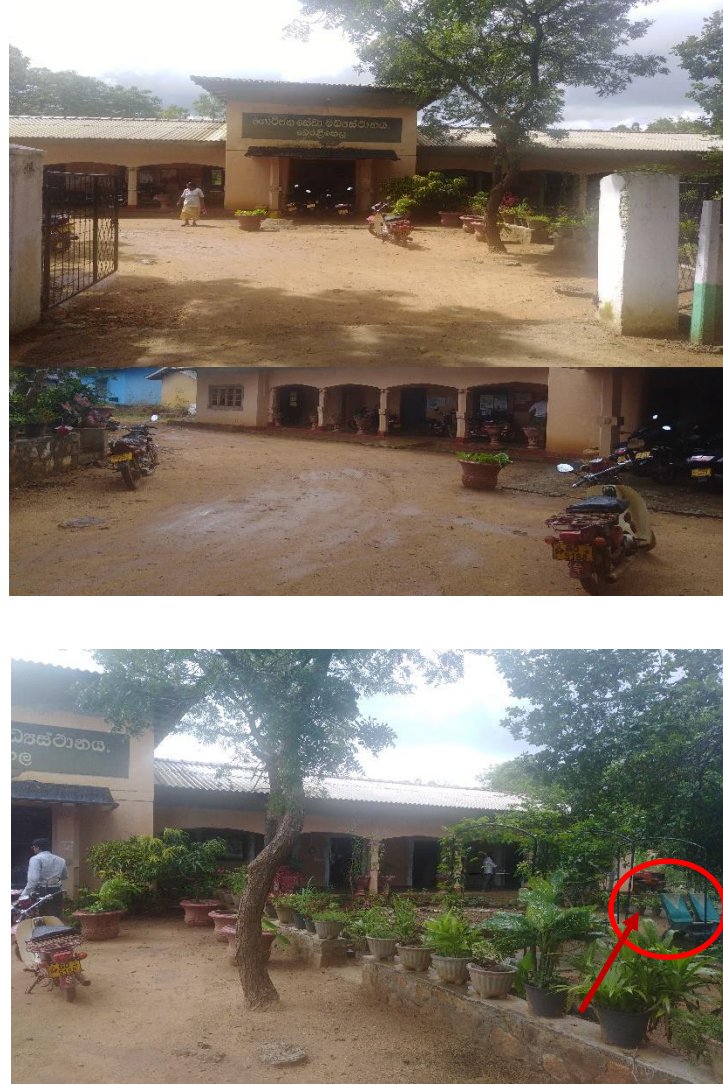
The building corner of the photo is to be built in the new section
